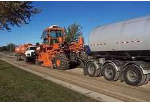
Expanded Asphalt Stabilization
