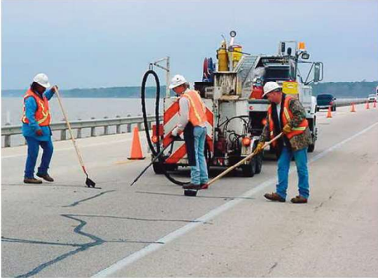
Crack Sealing
